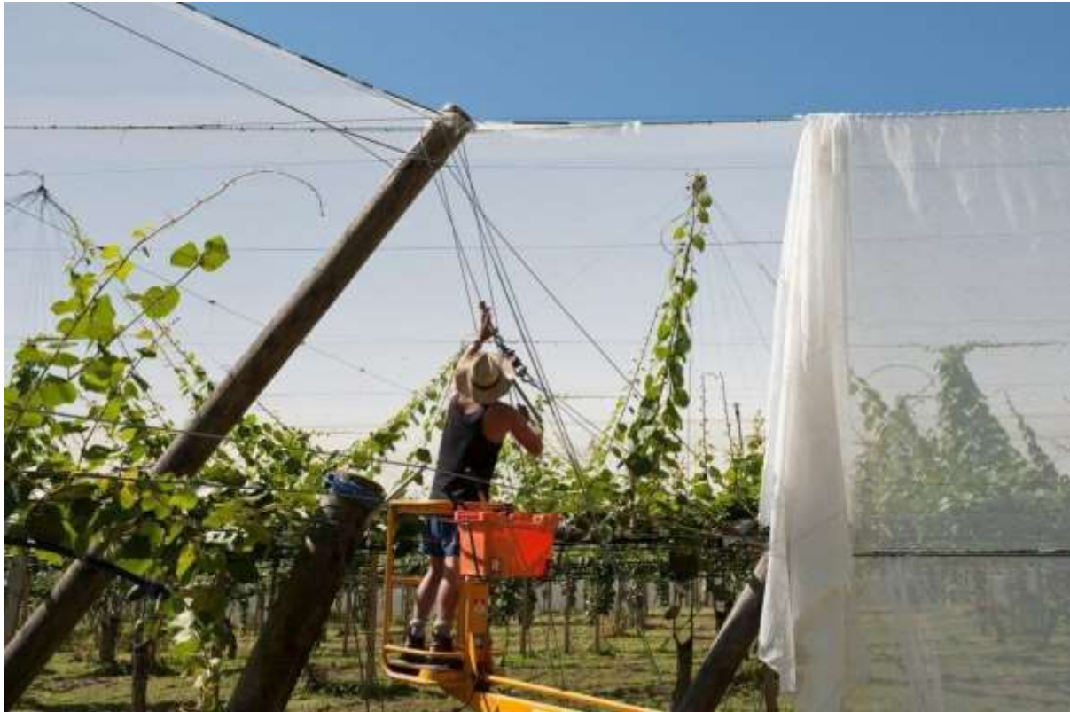
Image 20: The erection of hail netting over an orchard. In this instance the structure also has enclosed sides.
